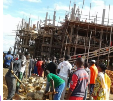
Building a technical school / Construction d'une école technique
